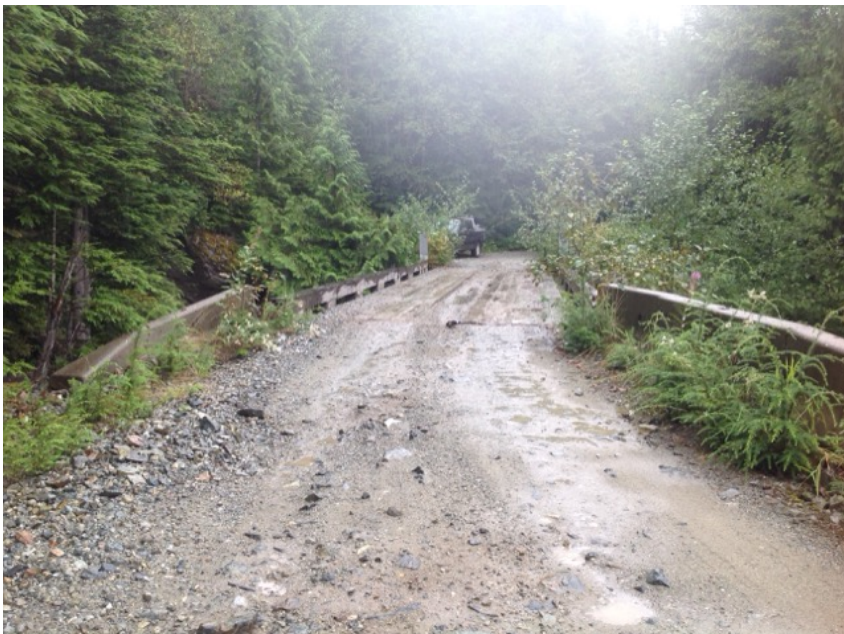
Approach from Right Bank when facing downstream
