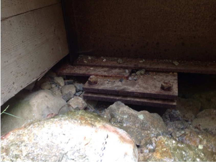
left upstream bearing
