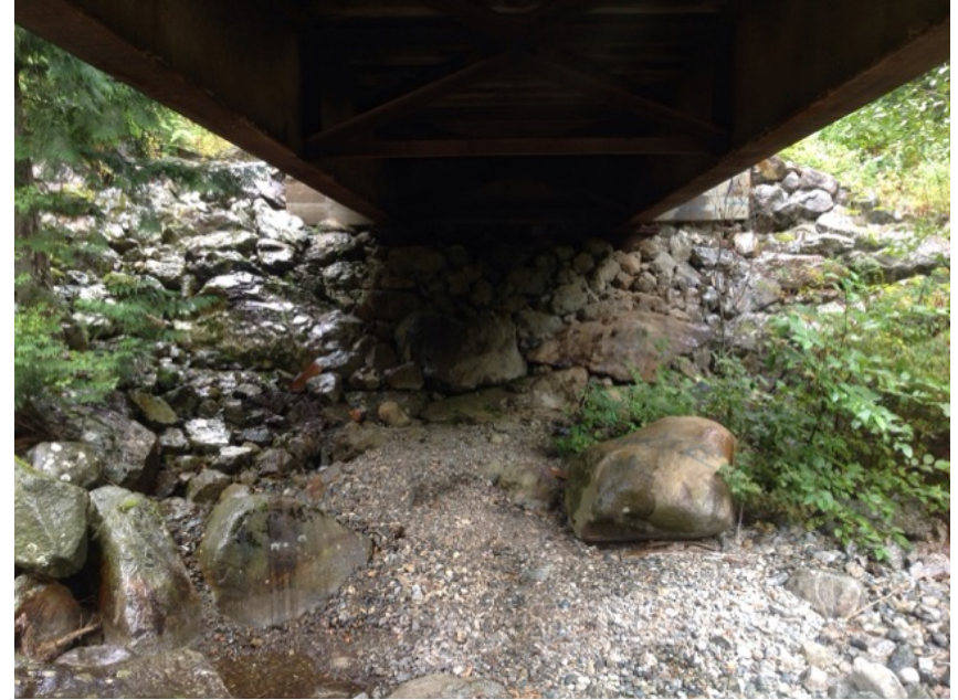
Left Bank Abutment when facing downstream
