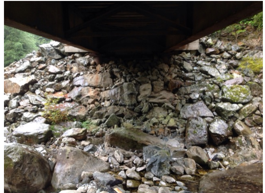
Right Bank Abutment when facing downstream
